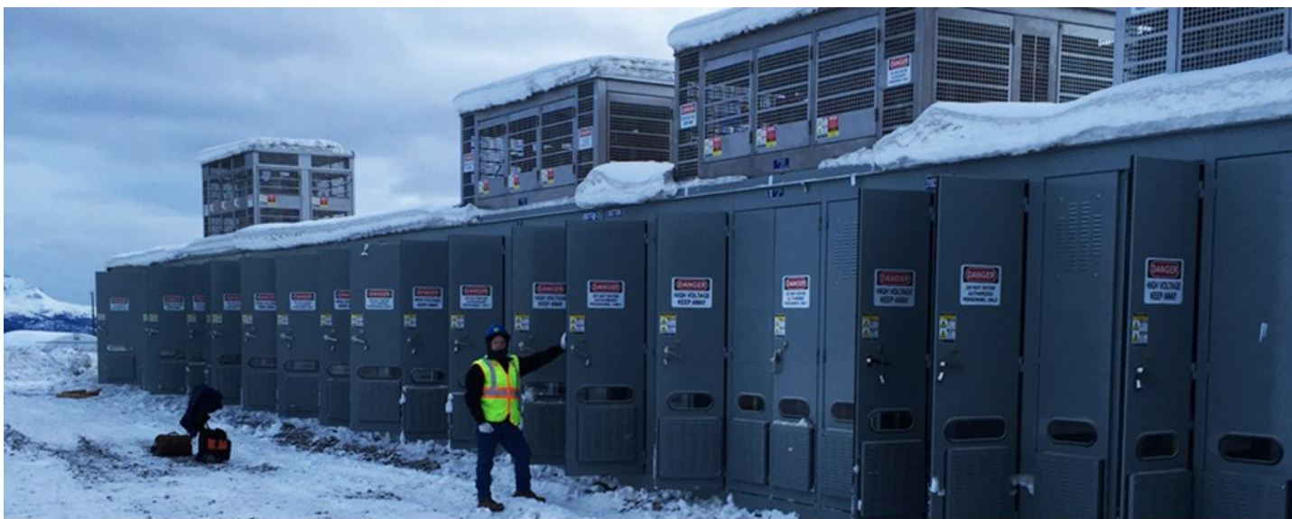
RED CHRIS MINE - BRITISH COLUMBIA C-High Pass, High Pass, and Notch Filter Branches 23 MVAR, 24.9 kV, 5-Stage, All-Inclusive Harmonic Filter System
